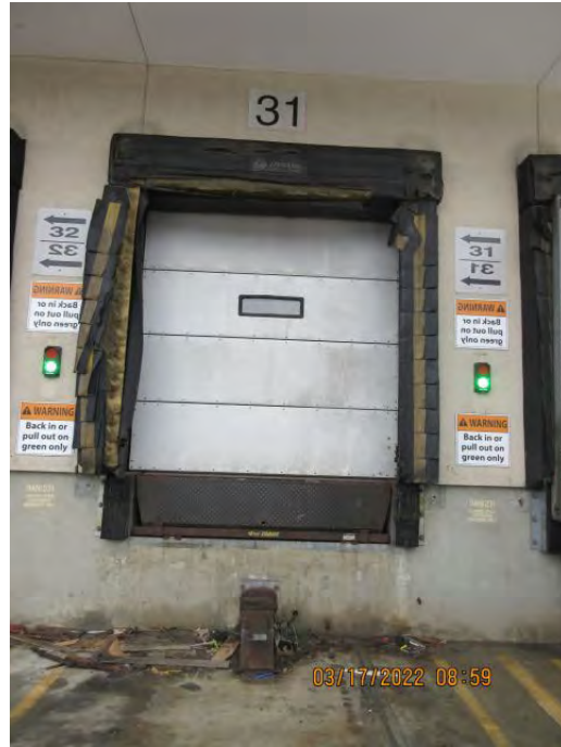
DOOR 31 Install Star 4 Truck Restraint
