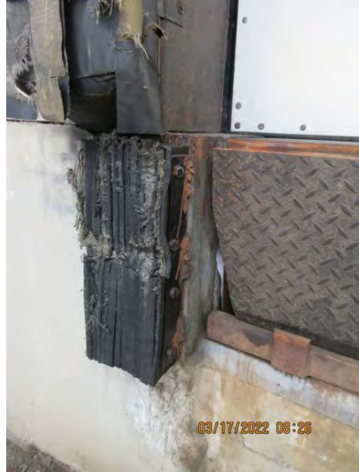
DOOR 22 Provide and Replace Rubber Dock Bumper
