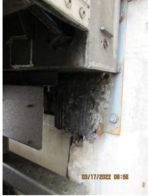
DOOR 30 Provide and Replace Rubber Dock Bumper
