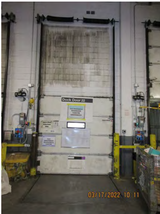
DOOR 22 Remove Existing Red/Green Light System
