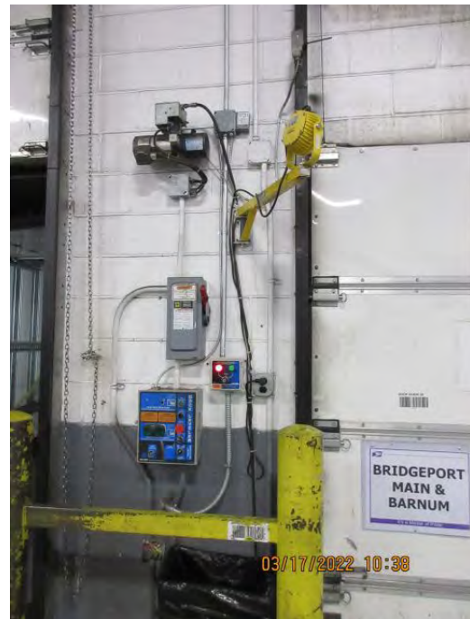
Existing Red/Green Light Controls, Left side of DOOR 28
