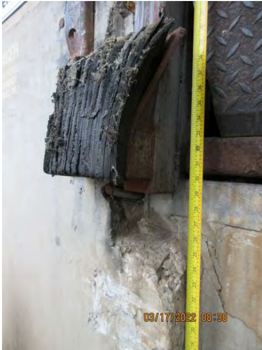
DOOR 25 Repair Spalling Concrete
