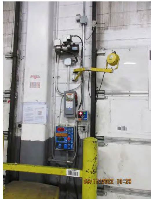
Existing Red/Green Light Controls, Left side of DOOR 26
