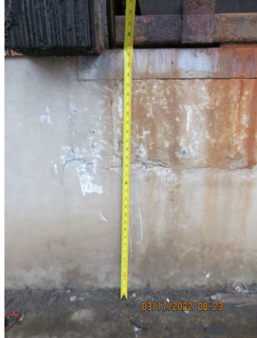
DOOR 21 Repair Spalling Concrete
