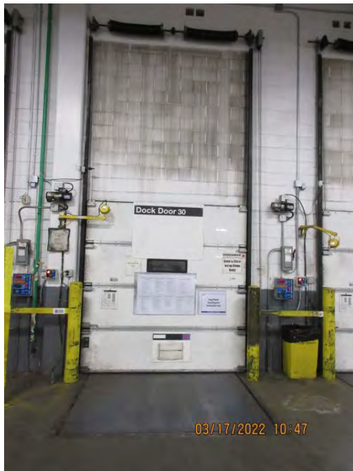
DOOR 30 Remove Existing Red/Green Light System
