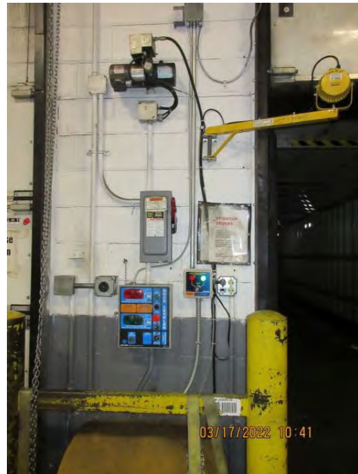
Existing Red/Green Light Controls, Left side of DOOR 29
