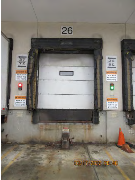
DOOR 26 Remove Existing TRS and Install Star 4 Truck Restraint
