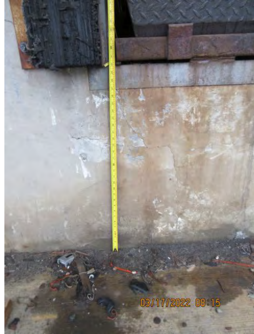
DOOR 19 Repair Spalling Concrete
