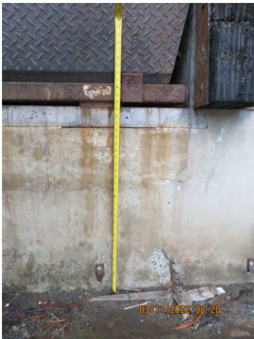
DOOR 22 Repair Spalling Concrete
