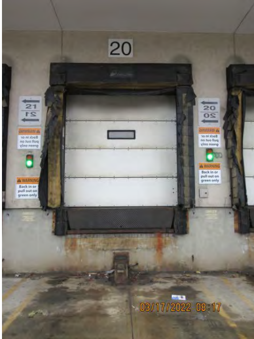
DOOR 20 Remove Existing TRS and Install Star 4 Truck Restraint
