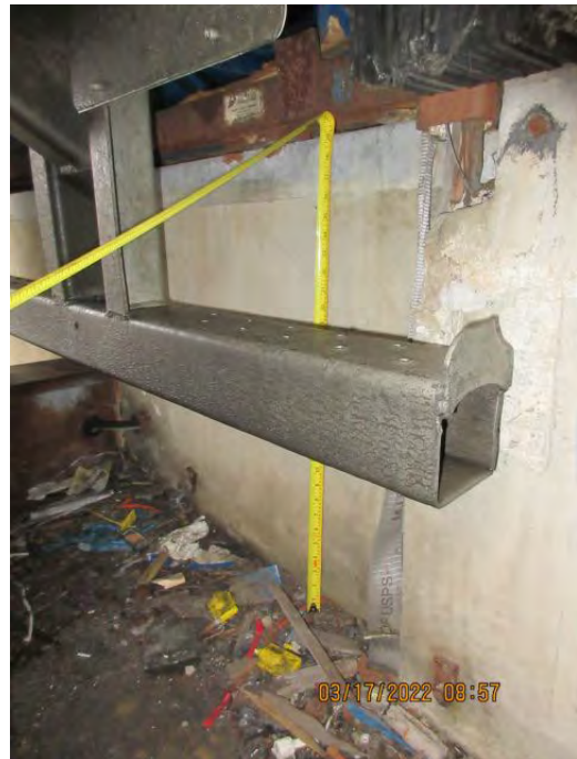
DOOR 30 Repair Spalling Concrete
