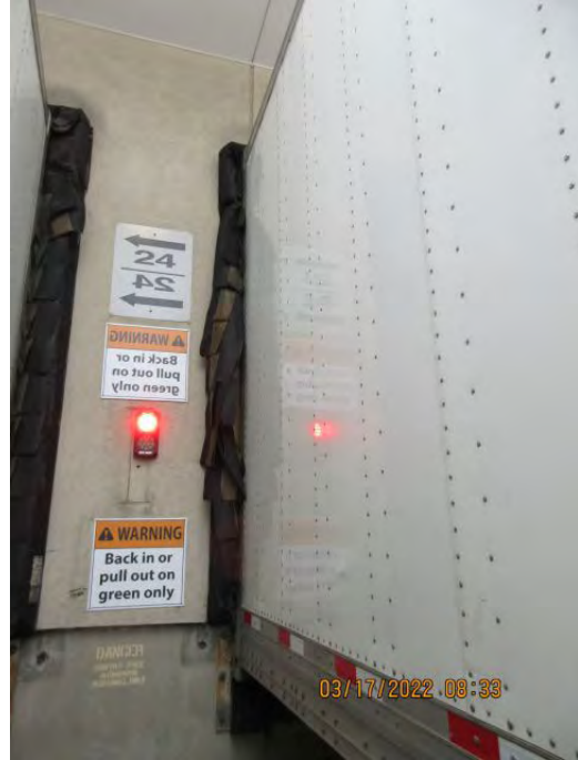
DOOR 24 Install Star 4 Truck Restraint
