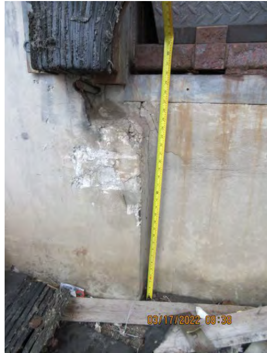
DOOR 25 Repair Spalling Concrete
