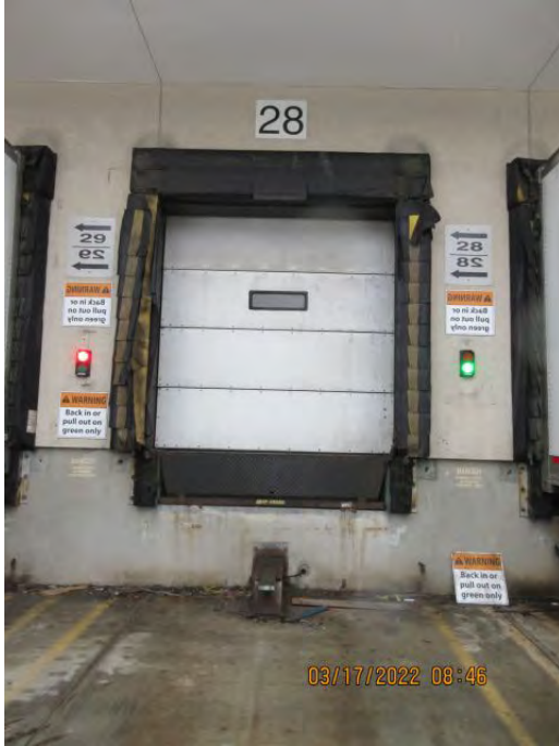
DOOR 28 Remove Existing TRS and Install Star 4 Truck Restraint
