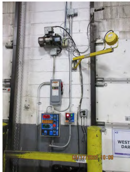
Existing Red/Green Light Controls, Left side of DOOR 21
