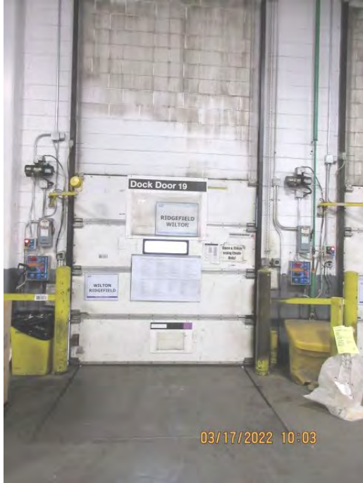
DOOR 19 Remove Existing TRS and Install Star 4 Truck Restraint
