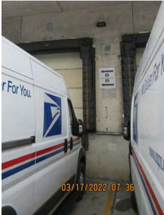
DOOR 8 Install Kelley Dock Communication System
