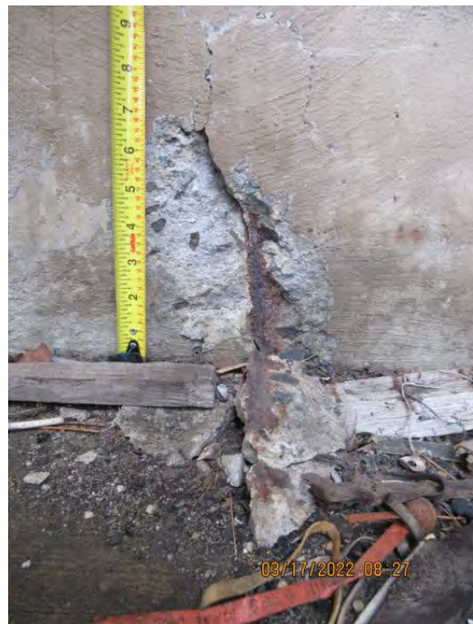
DOOR 22 Repair Spalling Concrete
