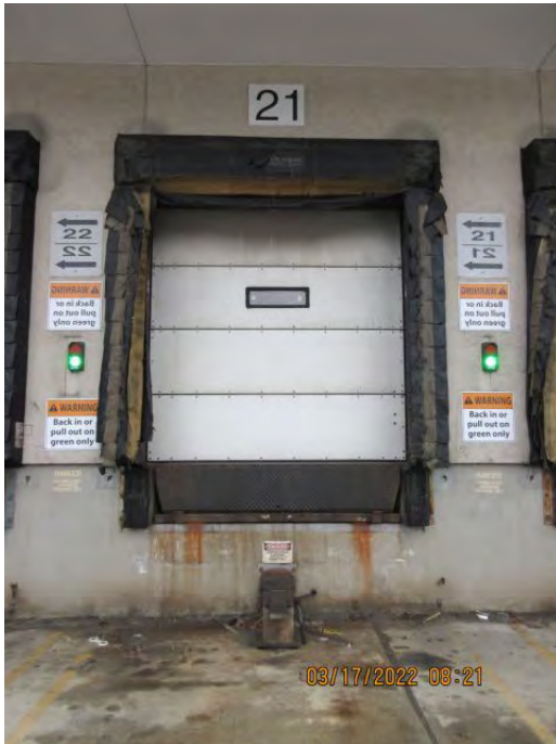
DOOR 21 Remove Existing TRS and Install Star 4 Truck Restraint
