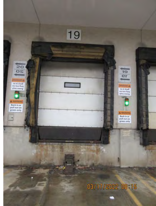
DOOR 19 Provide and Replace Rubber Dock Bumper
