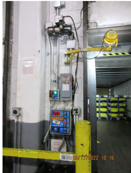
Existing Red/Green Light Controls, Left side of DOOR 23
