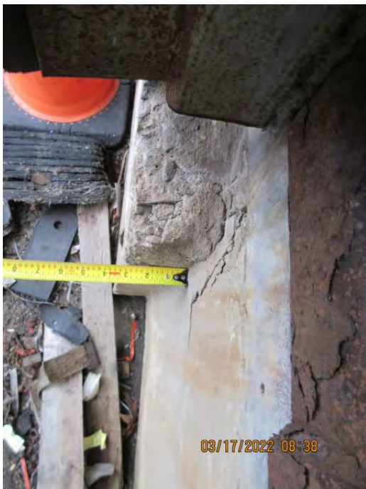
DOOR 25 Repair Spalling Concrete
