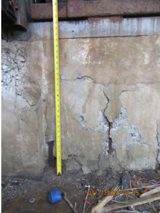
DOOR 22 Repair Spalling Concrete
